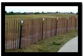
The snow fence application was used on this site because winds were a significant issue. There are two, four-foot wide pieces of poultry wire where one is laid on the ground to discourage prairie dogs from digging under the barrier. The other piece applied vertically discourages prairie dogs from going through the wood slats.
