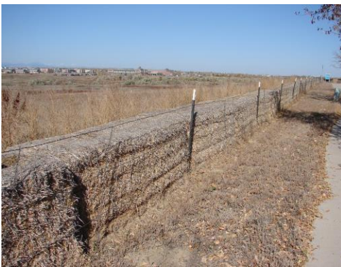
Straw bales along prairie dog side of fencing.
