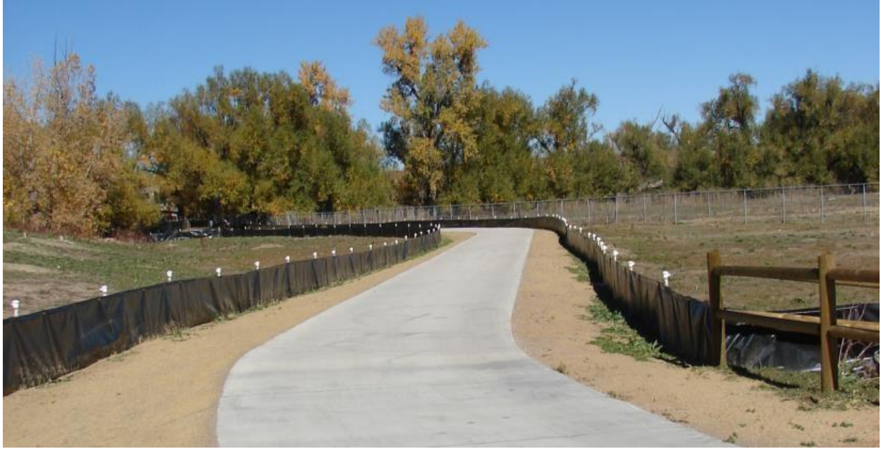
Temporary vinyl barrier used during construction project.
