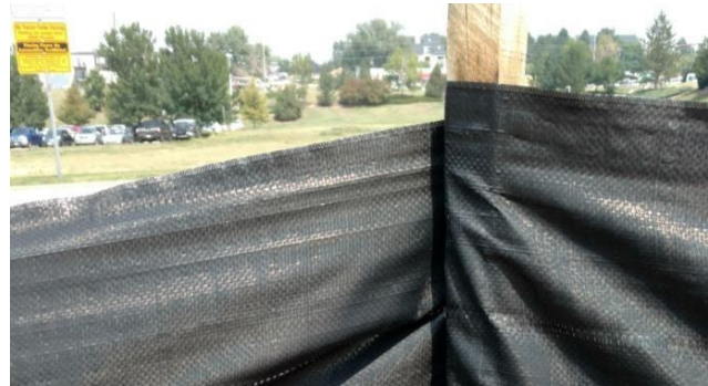
Modification: Twist fabric around stake for longevity
