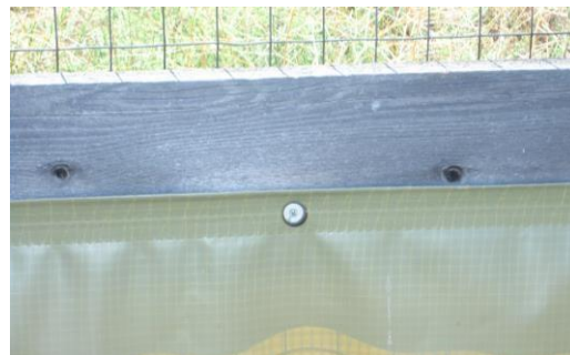
Screw and washer through grommet
