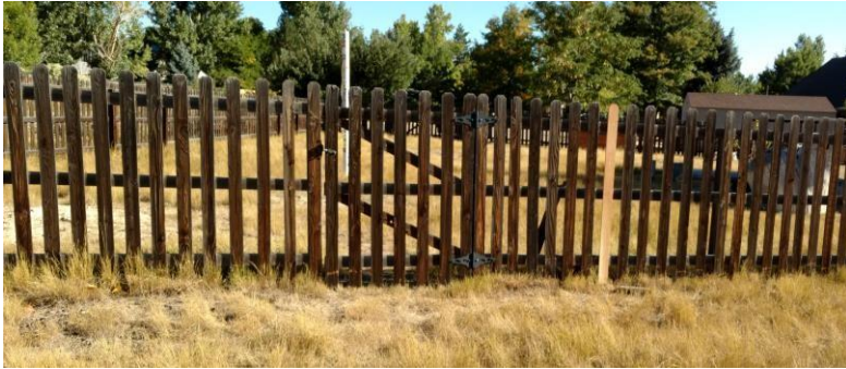
Existing fence before modification
