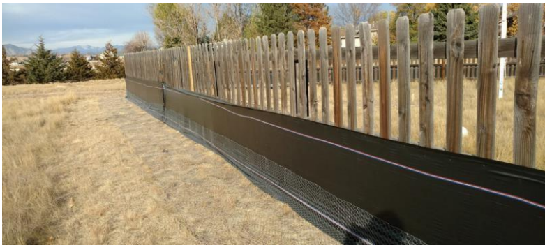
Modified to exclude prairie dogs by adding black silt fence and skirting.
