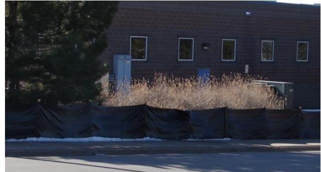
Silt fence used for pending construction.
