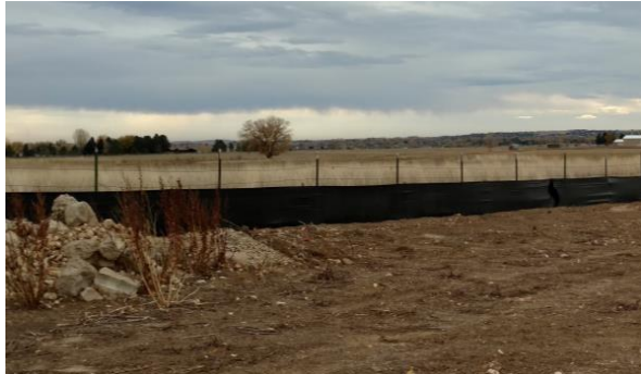
Silt fence used in large field
